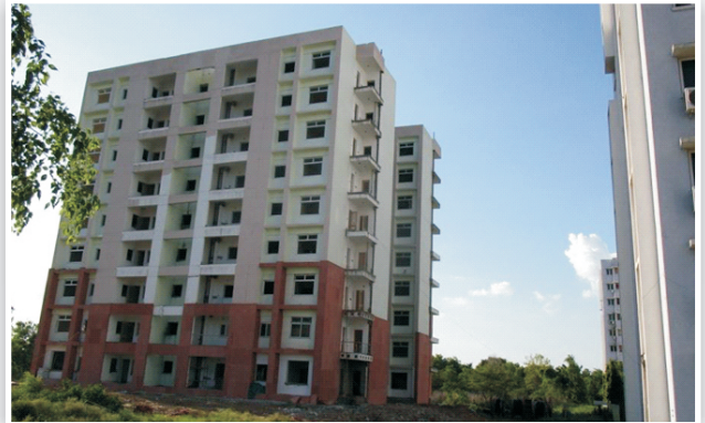
B type quarters work is in progress
