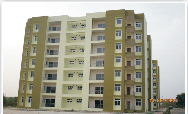
C type quarters completed
