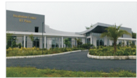
Fig 4.: 30,000 Sq Ft Permanent Facility
