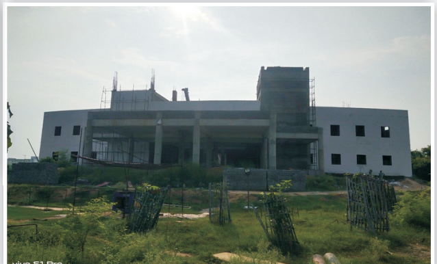
Auditorium building work is in progress
