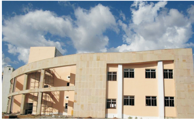
Lecture hall work is in progress
