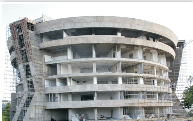
Library building work is in progress
