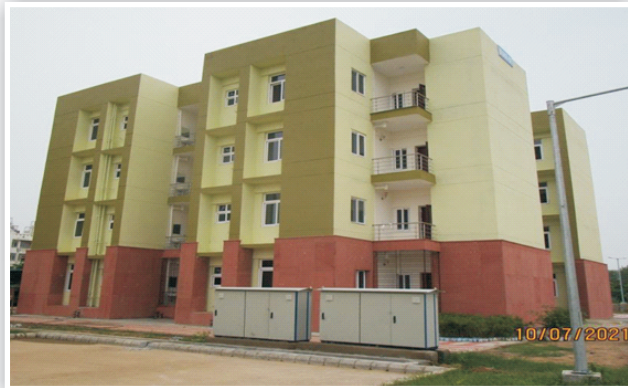
D type building completed
