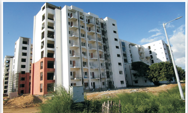
Boy's Hostel work is in progress
