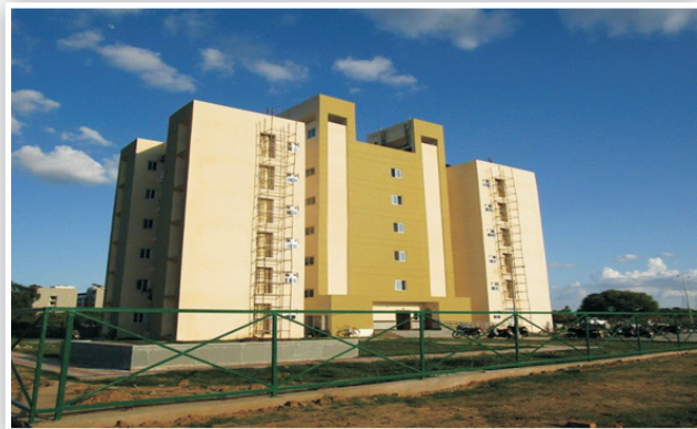
Married Accommodation completed
