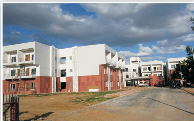
Guest house almost completed
