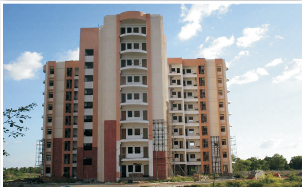
A type quarters work is in progress
